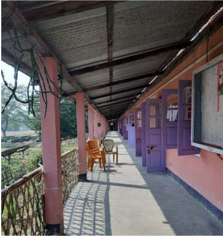
A view of College Verandah
